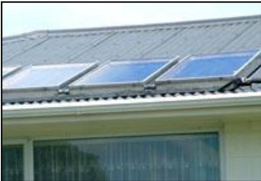
Solar water-heating panels can be metal or plastic, fitted onto or into the roof, and are usually glass-glazed, over either a black heat plate or a set of parallel glass tubes. Compare systems and ask for test results.
