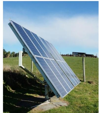
If your home is a long way from existing mains grid supply lines, investment in battery storage and a larger array of PV panels becomes cost-effective, as in this example photographed on a Canterbury farm: these panels are motorised to track the sun by day, increasing efficiency. Lower cost panels today make it sensible to buy a few extra but fix all at north orientation, without tracking machinery.
