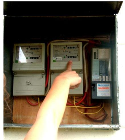
Reading the electricity meter. The numbers displayed usually include tenths of a kWh unit, at the right. There's no requirement here for accuracy down to tenths of a unit, but be consistent if you do record figures below the decimal point, or your use calculations could be out x10.
