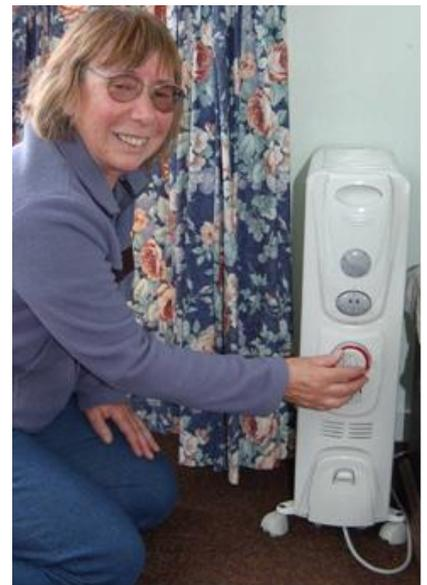
**Setting a timer** on an oil-filled radiator. This one has an adjustable thermostat and option of two levels of heat input.
